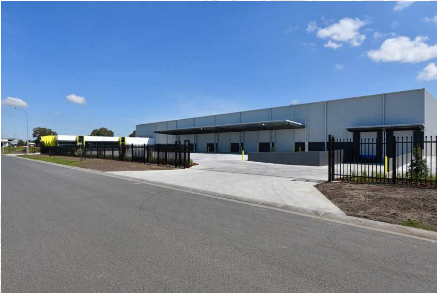
New ETD/Dynamic warehouse Dandenong Vic.
